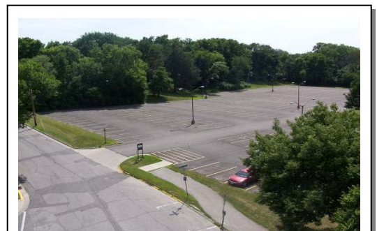
LOT 60 - ORIGINAL CONDITION
