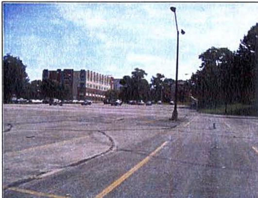
PHOTO 9: FACING EAST AT SUBJECT PARKING AREA FROM EDGE OF PARKING LOT
