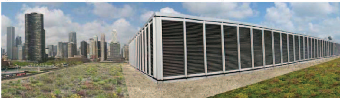
Jardine Water Purification Plant - Extensive System
