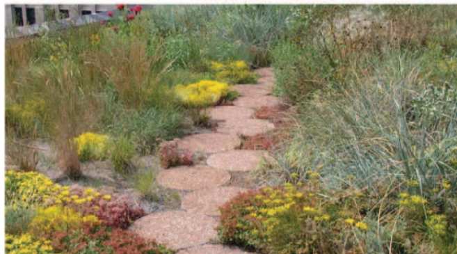
Chicago City Hall Green Roof - Semi-Intensive System
